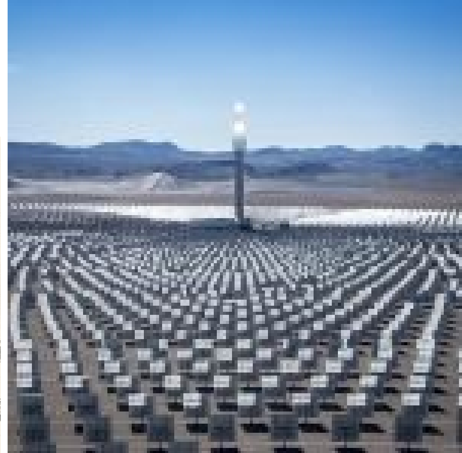
Crescent Dunes solar thermal
